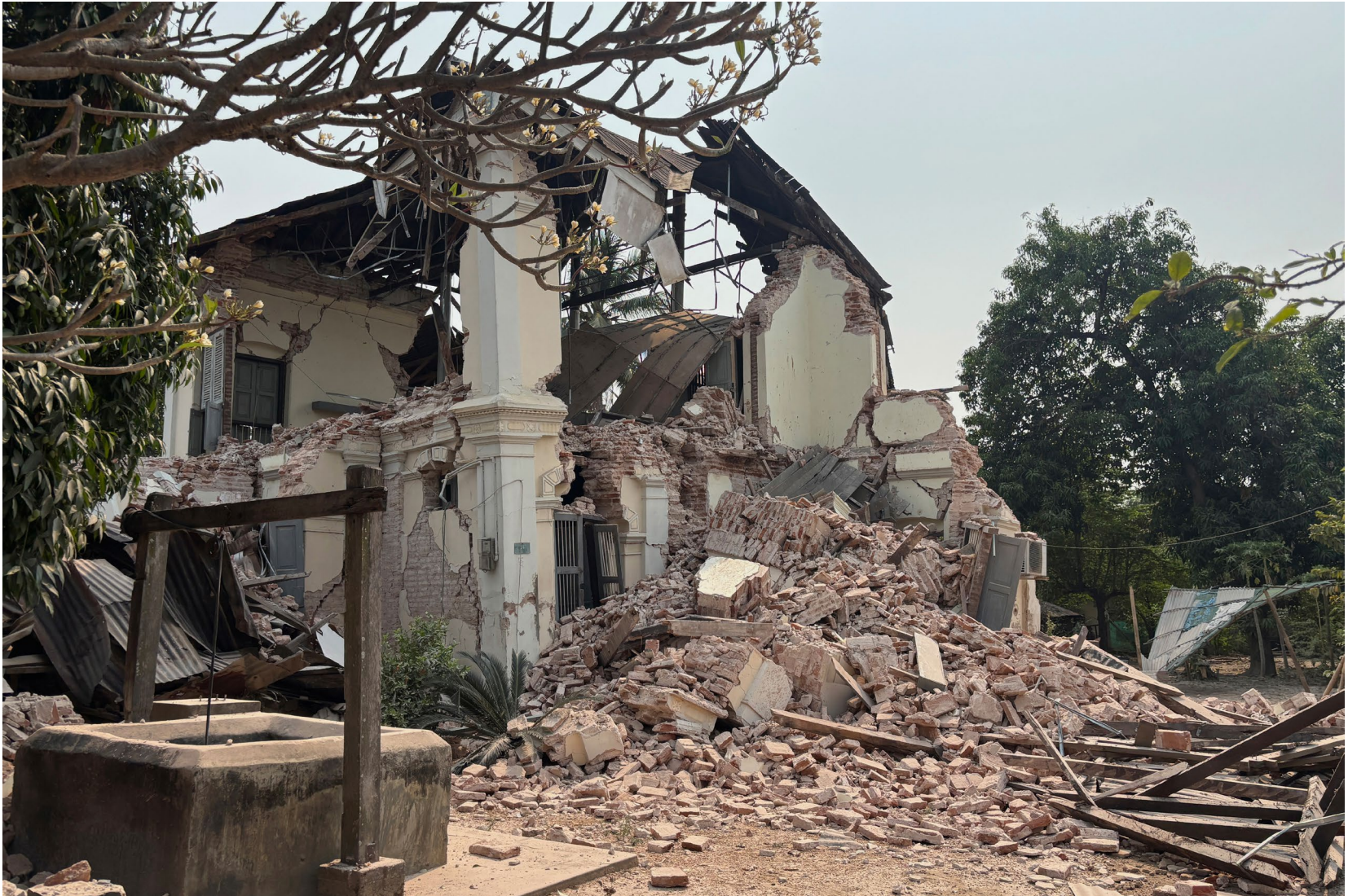
A building is damaged after earthquake Friday, March 28, 2025, in Nay Pyi Taw, Myanmar. (AP Photo/Aung Shine Oo)
